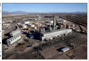
At the H. Wilson Sundt Generating Station, power is generated by two gas turbines and four steam turbines ranging from 83 to 165 megawatts. The steam units can be fueled by coal, natural gas, or fuel oil. In addition, landfill gas from Los Reales landfill is used. Generally, though, about 90% of the power generated at the station is from coal.
